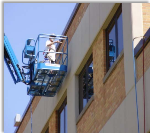
Exterior wall repairs at Ellsworth AFB, SD
